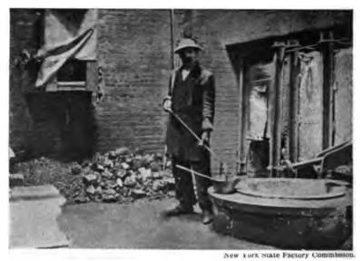
Lead Refining. Pot of Lead Drawn from the "Sweater" from which the Caster is Ladling Molten Lead.
